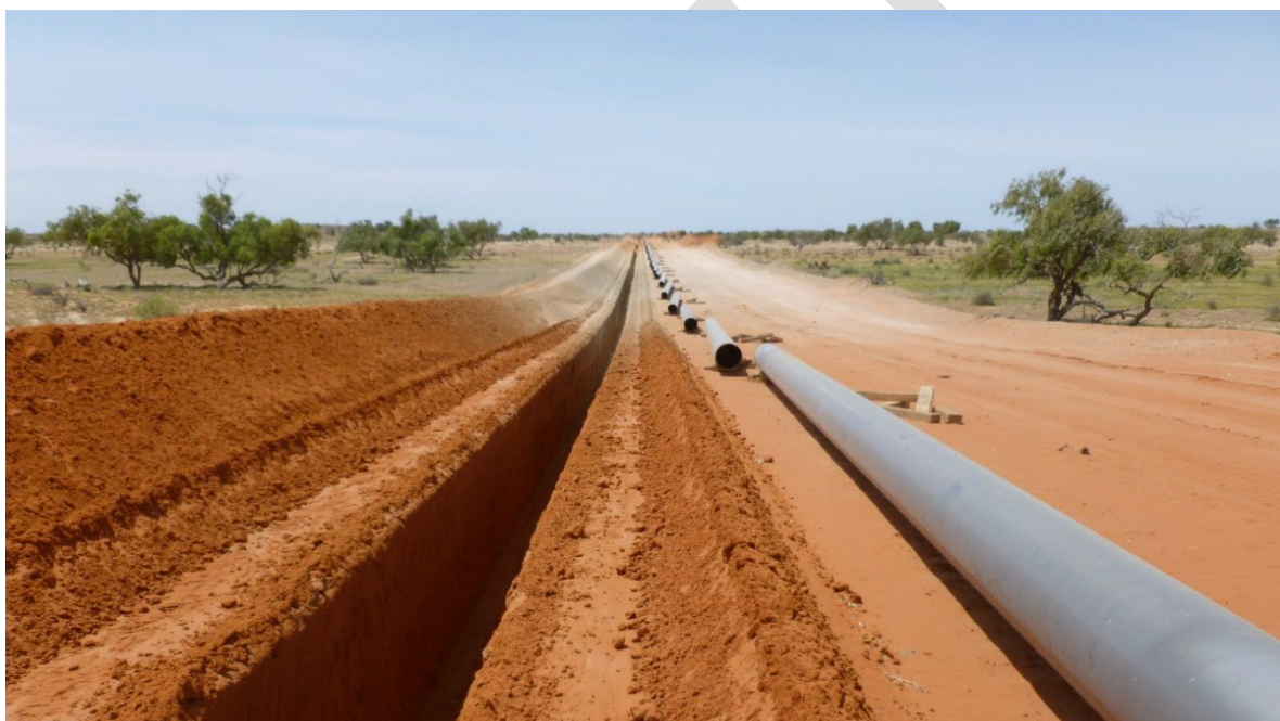
Plate 3-1: Example of pipe stringing
