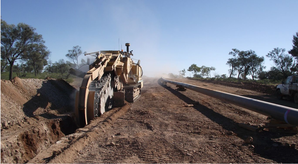
Plate 3-2: Example of pipeline trenching
