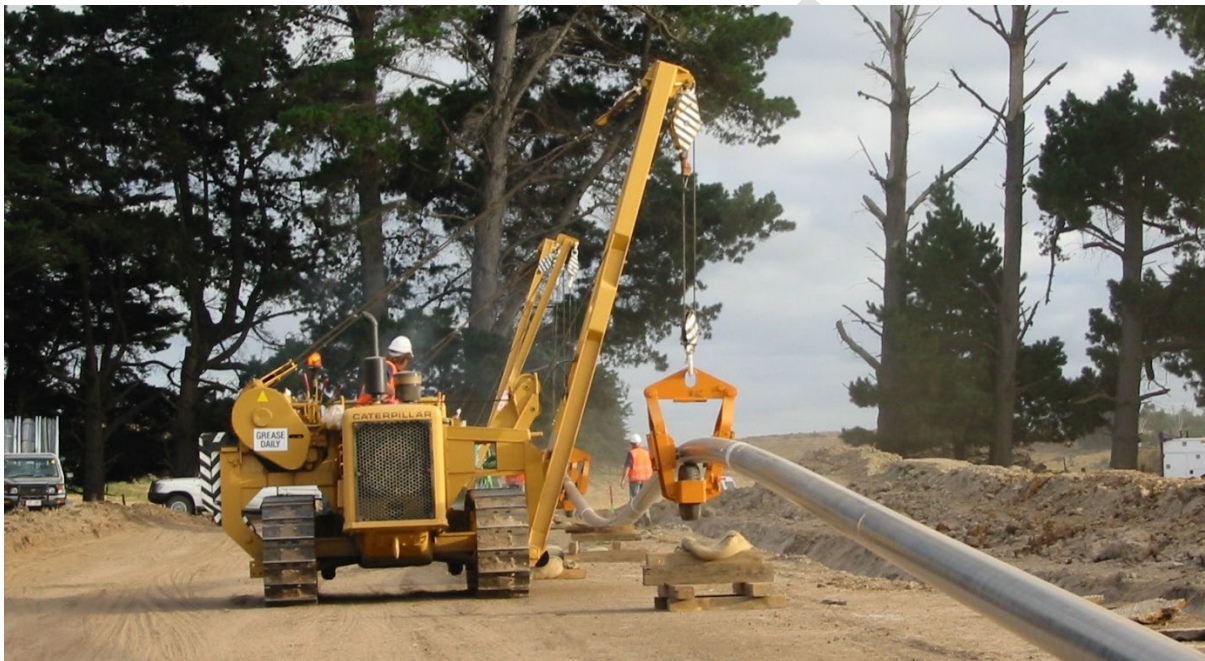
Plate 3-3: Example of pipeline lowering-in
