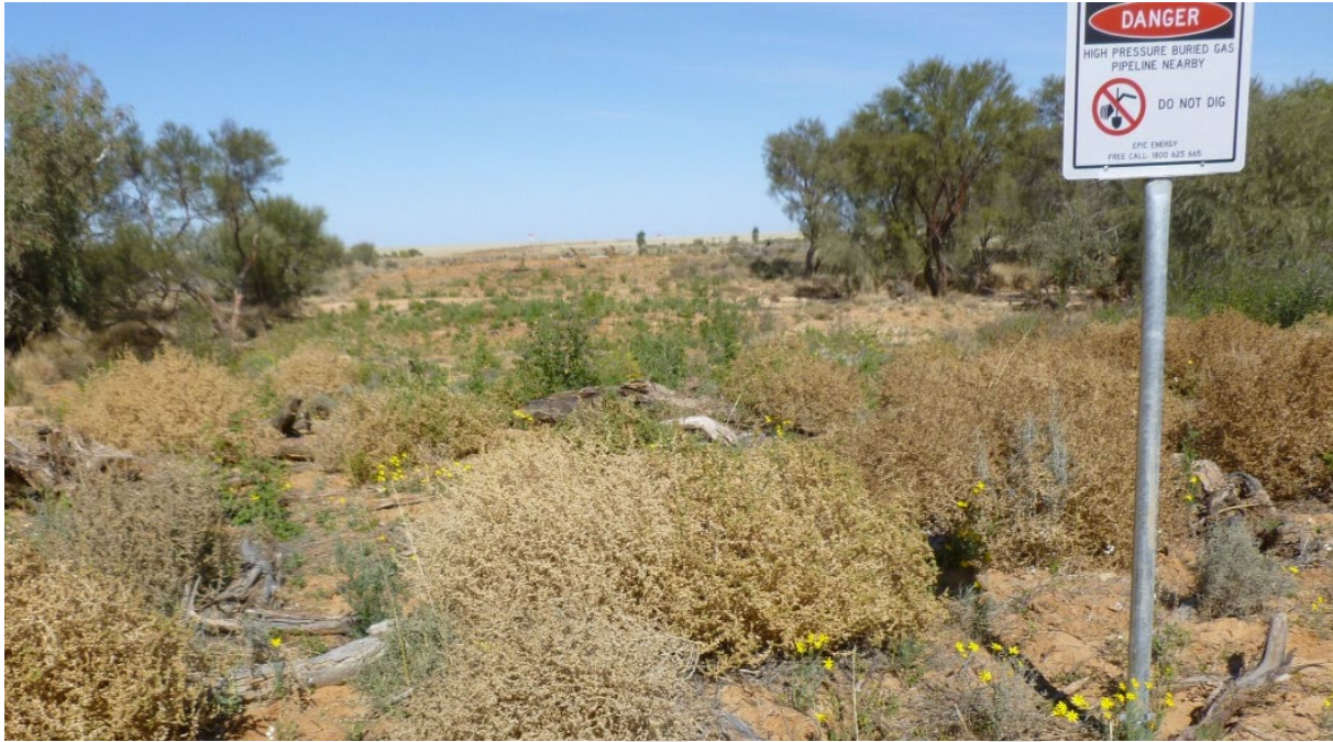
Plate 3-4: Example of rehabilitated right-of-way and marker post 12-18 months post construction (Epic Energy QSN3 pipeline)
