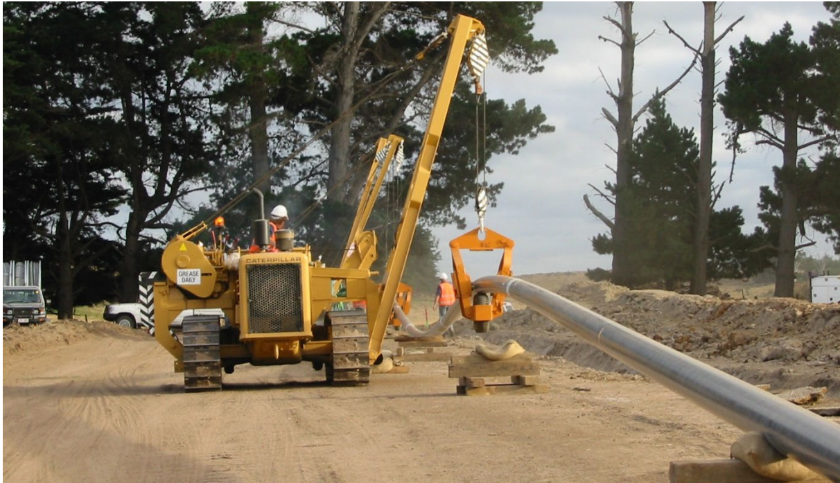
Plate 2-3: Example of pipeline lowering-in
