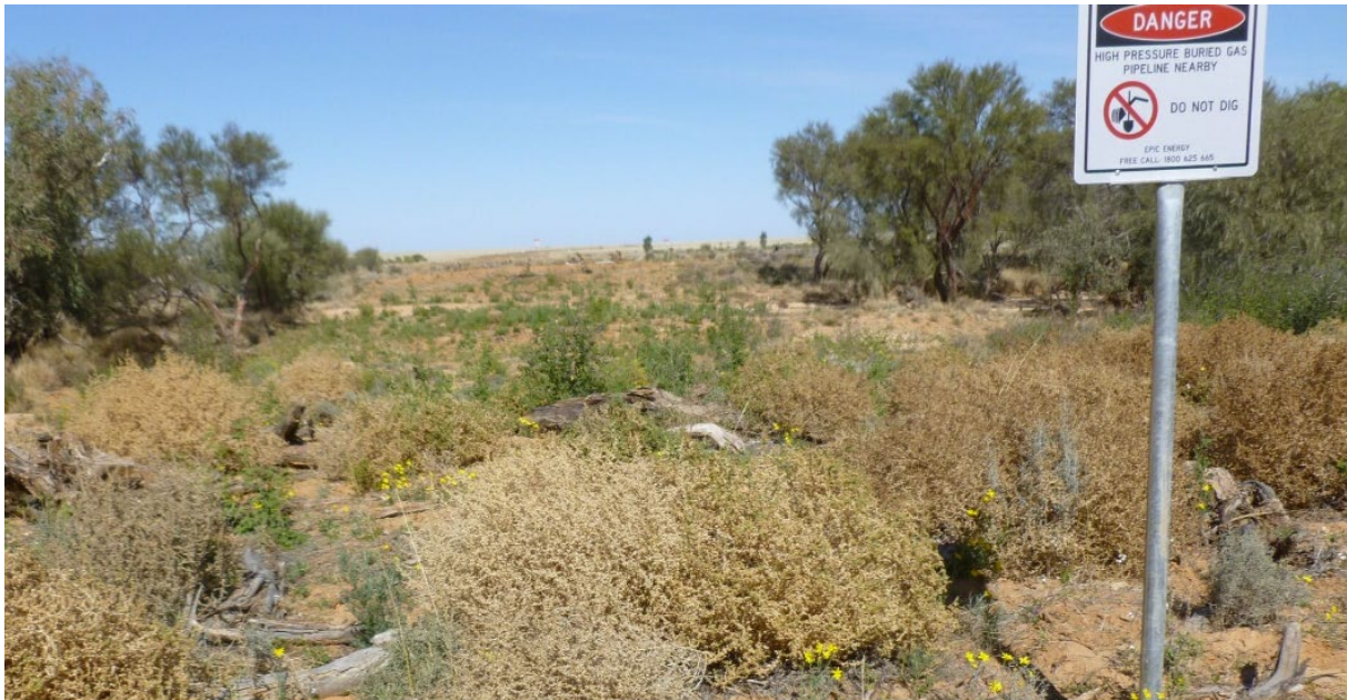
Plate 2-4: Example of rehabilitated right-of-way and marker post 12-18 months post construction (Epic Energy QSN3 pipeline)
