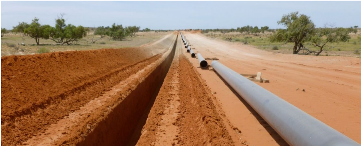
Plate 2-1: Example of pipe stringing
