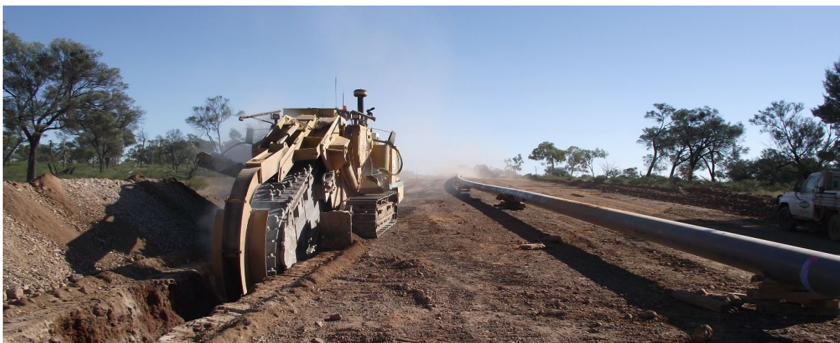
Plate 2-2: Example of pipeline trenching
